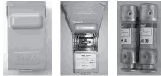
Disconnect switch box for outdoor unit
